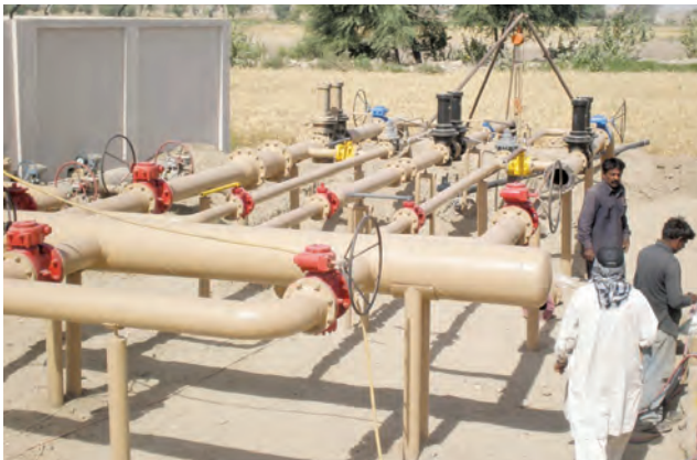
Segregation work in progress at Sarhari and Padidan SMSs
